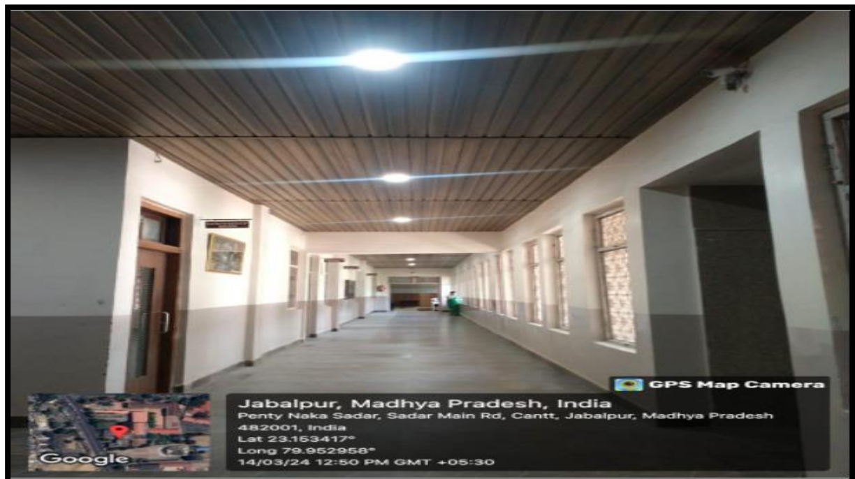
View of Corridor
